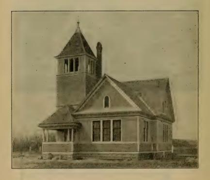
Church at Vesper, Kansas. This is a peculiarly neat and conveniently arranged building—the two rooms opening into each other so that all can be used together. The floor of the Sunday-school room is raised 18 inches above the floor of the main room. The cost was about \$2,500. For ground plan see next page.
